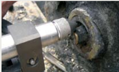
Installation of cutting device
