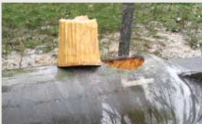
Cutting an access hole
