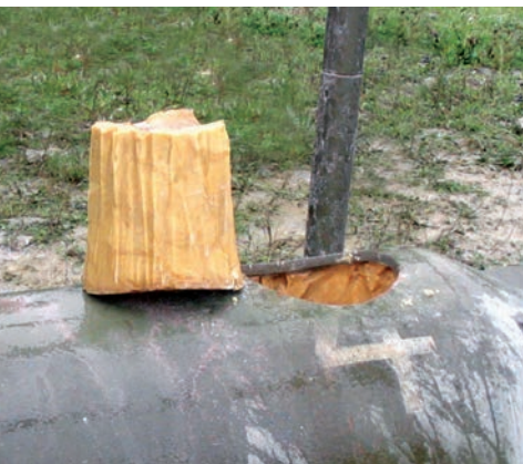
Cutting an access hole (in explosives)
