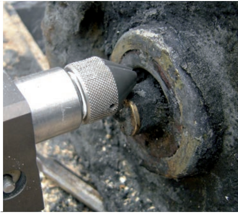
Installation of cutting device
