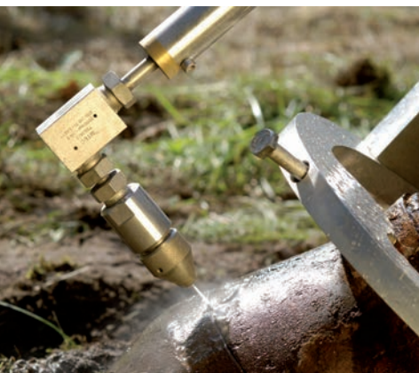
Cutting with Base Fuse Manipulator
